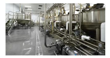
Like all urethane cements, it is necessary to honor the joints. Diamond-FJF urethane joint filler is recommended.
